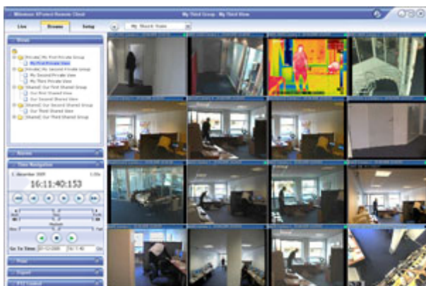
Example of the Remote Client, displaying video from 16 cameras
